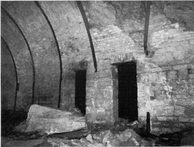
Brickwork and cast iron lining (B on the plan).
